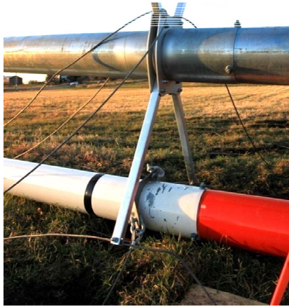
Picture 3-49: Threading the jumper strut cable
