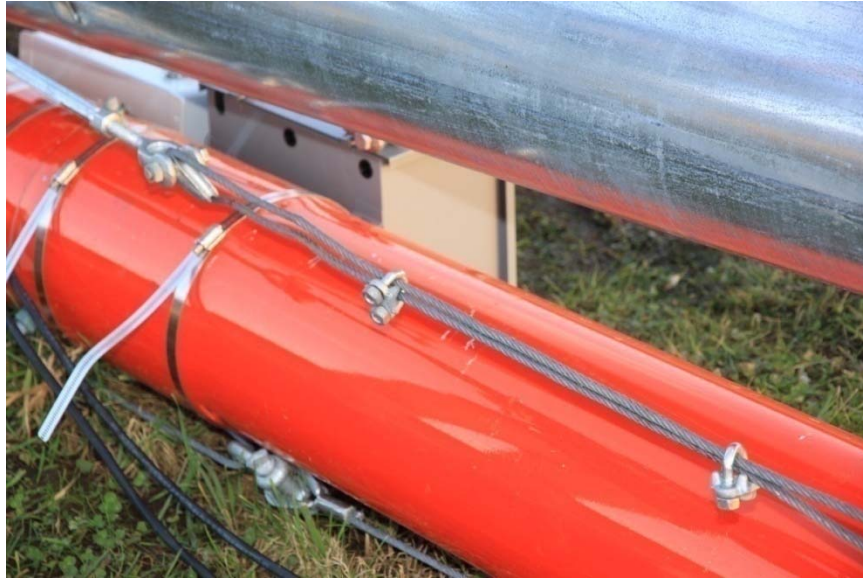
Picture 3-51: Attach jumper strut cable to turnbuckle
