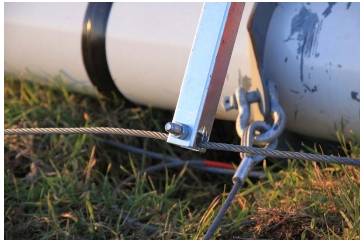
Picture 3-50: Threading the jumper strut cable
