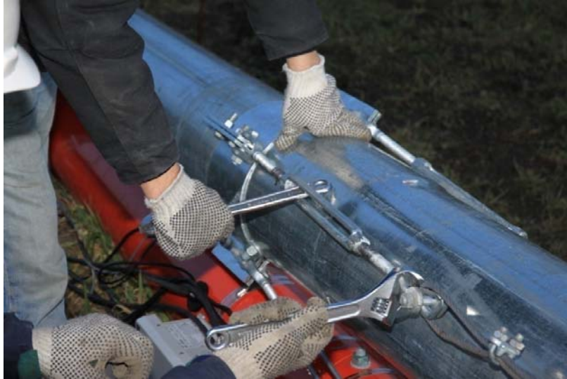
Picture 3-79: Tightening turnbuckles
