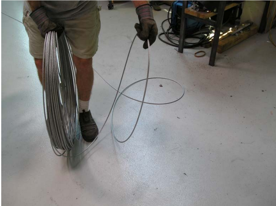
Picture 3-32: Unroll guy wires INCORRECT
