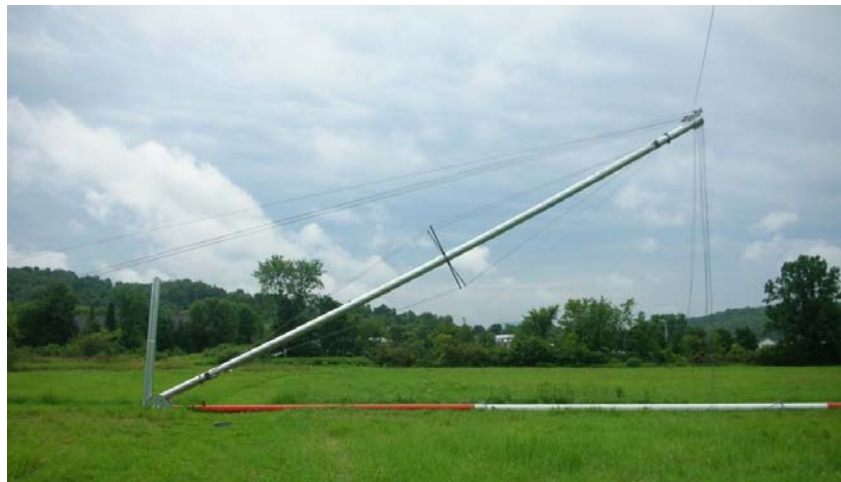
Picture 4-1: Correct time to check for winch cable twists-if all is good, remove the helper ginpole
