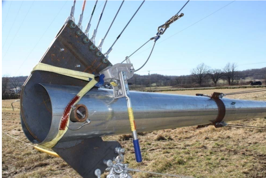
Picture 4-10: Set up for transferring lifters to their storage anchor
