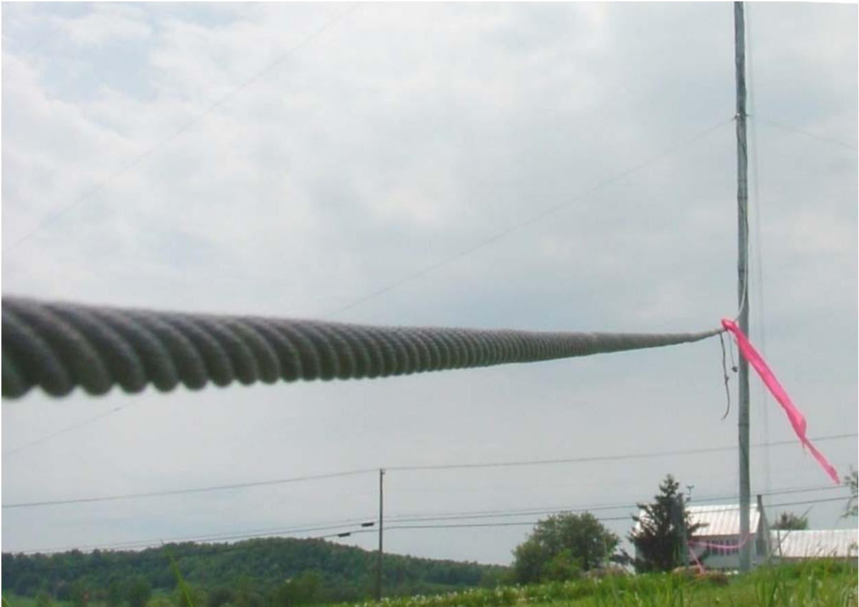
Picture 4-8: Level 1, guy sag = 2.5 tubes - too loose
