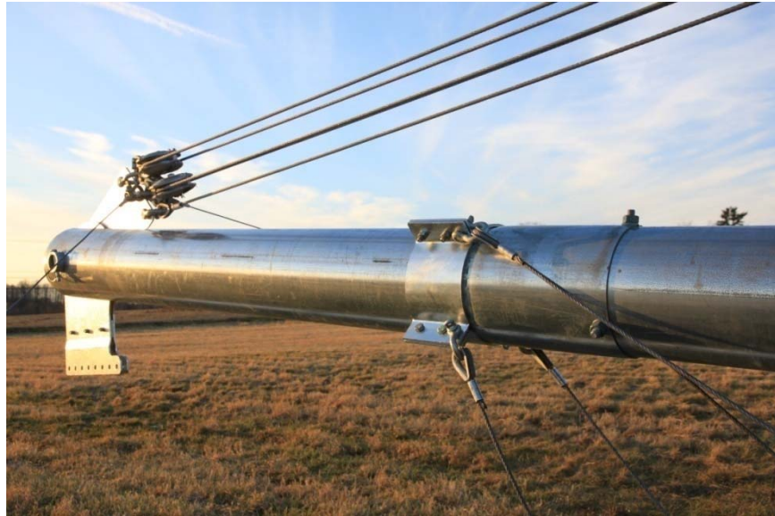
Picture 3-47: Jumper strut cable attachment
