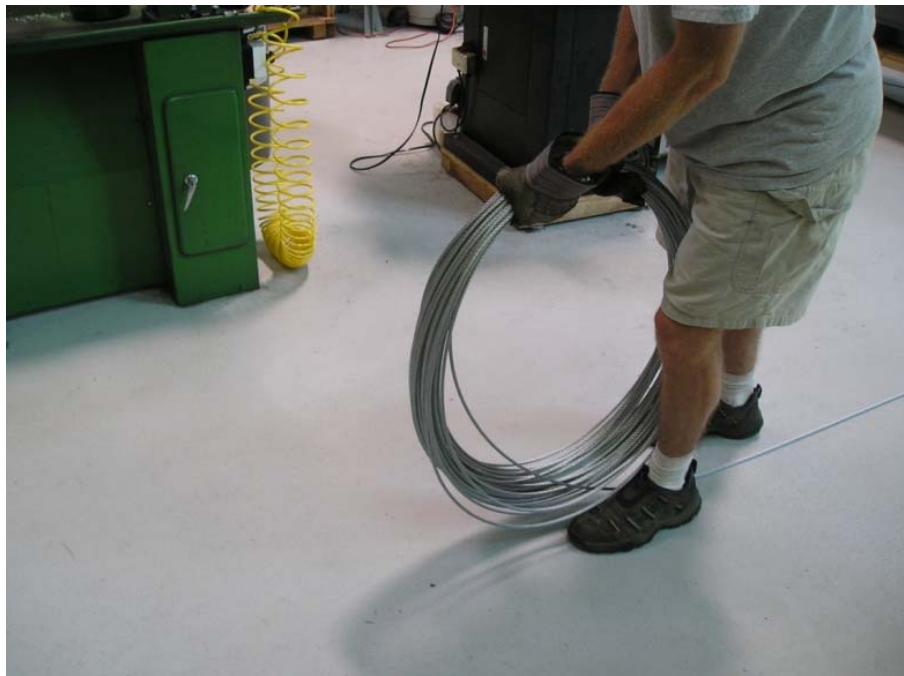
Picture 3-31: Unroll guy wires CORRECT
