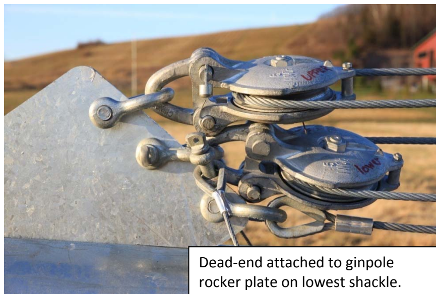
Picture 3-78: Affixing dead-end to ginpole rocker plate
