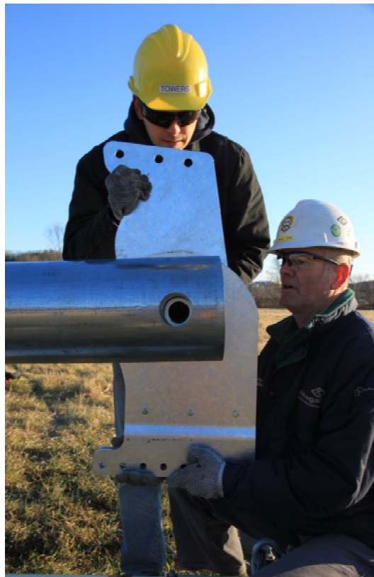
Picture 3-54: Ginpole rocker plate assembly
