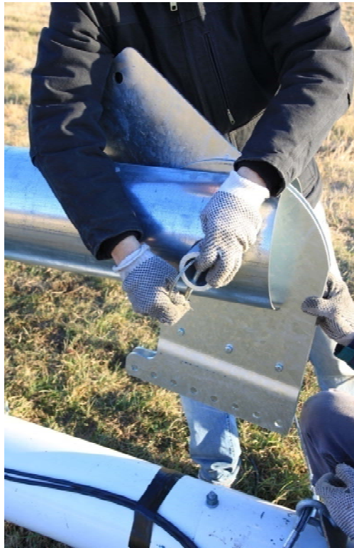
Picutre 3-55: Secure ginpole rocker plate pivot pipe
