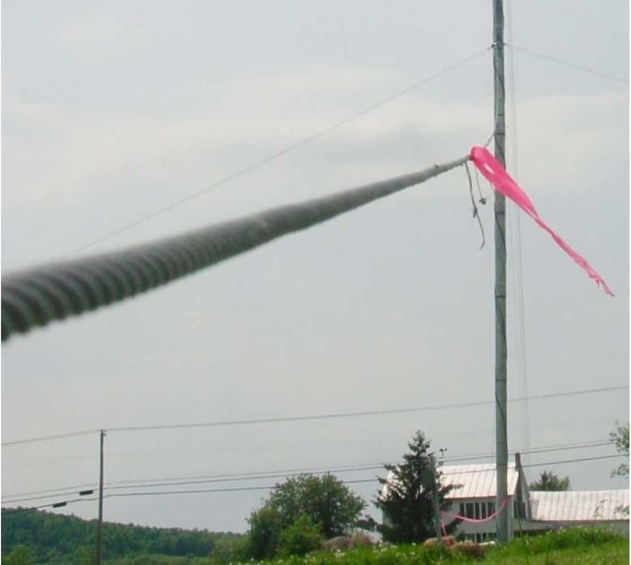
Picture 4-7: Level 1 guy, sag = 1-1/4 tube - just right
