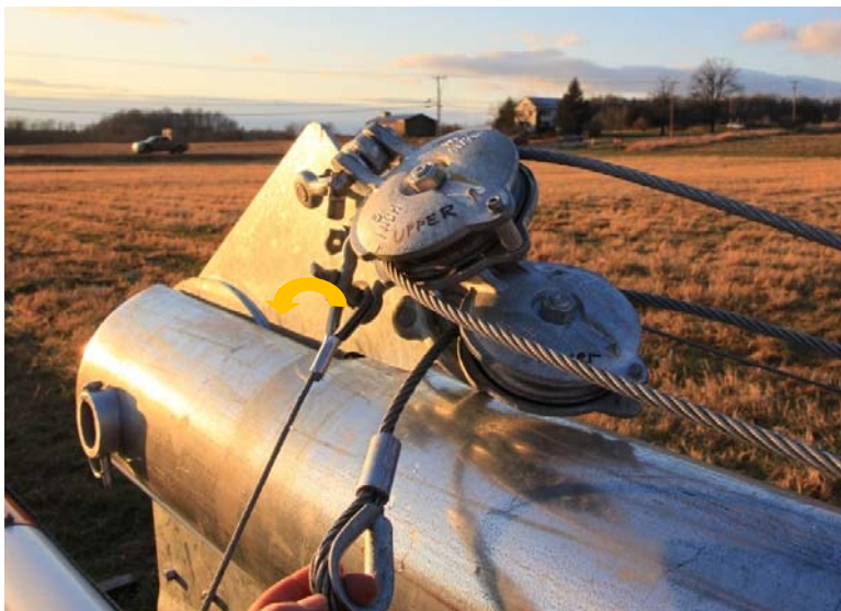
Picture 3-75: Reeving through pulley #4
