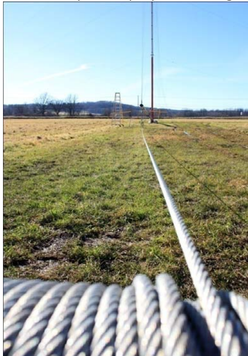
Picture 3-68: Correct winch cable fleet angle
