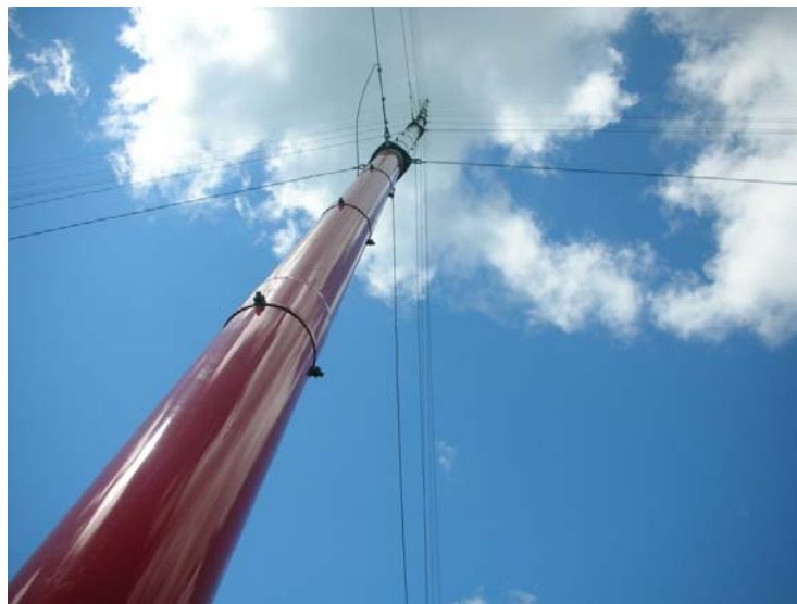
Picture 4-5: Straightening your tower
