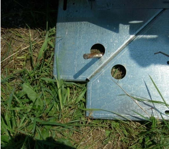
Picture 3-12: Ground Rod Placement
