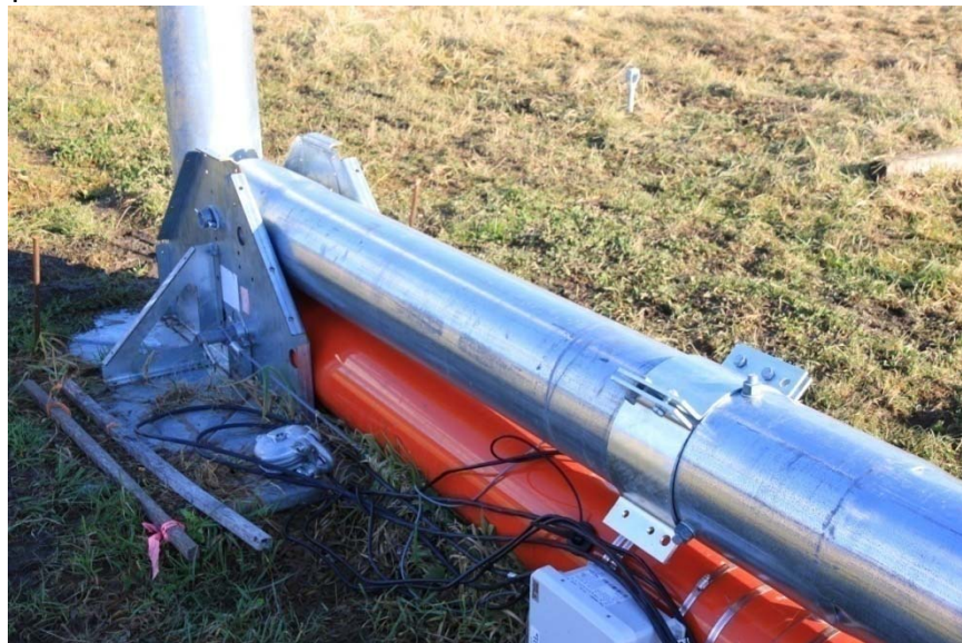
Picture 3-40: Ginpole jumper strut end-flanges
