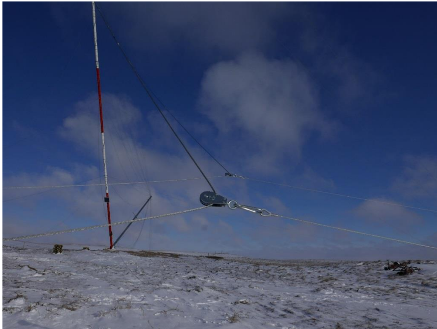
Picture E-4: Leader cables attached to back guywires using pulleys
