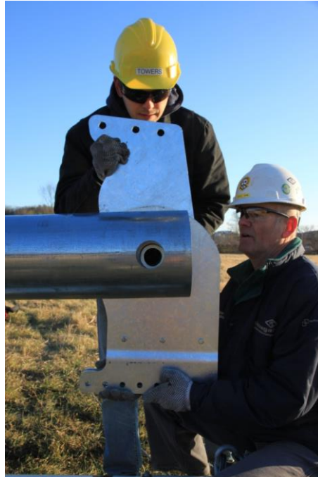
Picture 3-55: Ginpole rocker plate assembly
