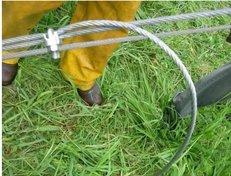
Picture 3-34: Wire rope clip guy wires together at anchor points
