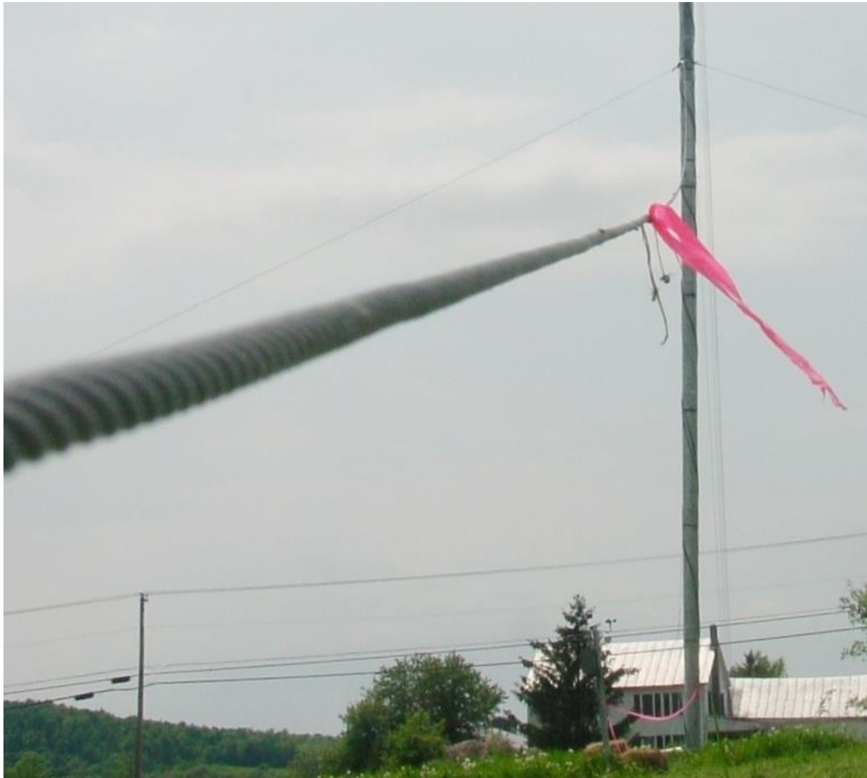
Picture 4-7: Level 1 guy, sag = 1-1/4 tube – JUST RIGHT!
