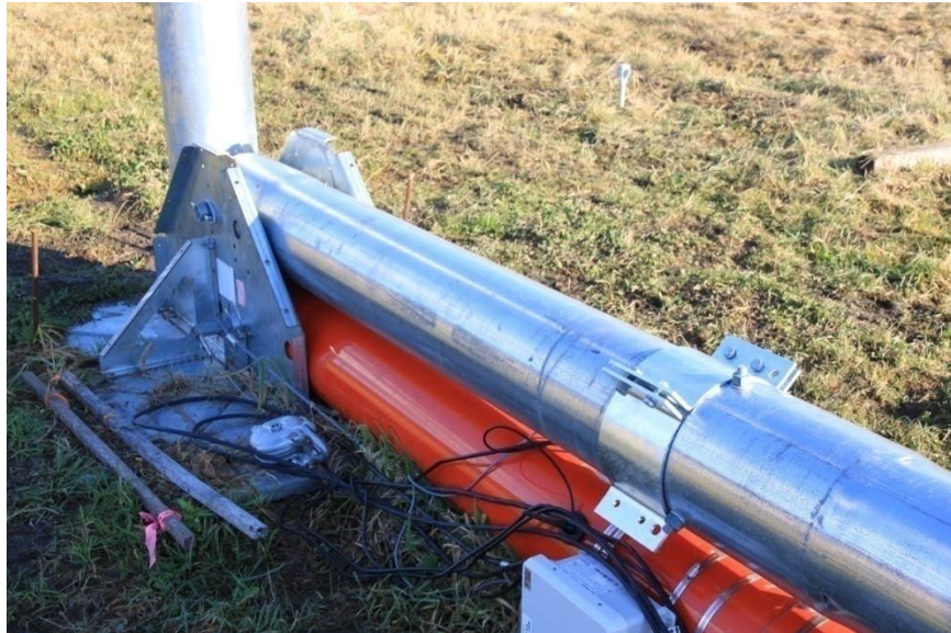
Picture 3-40: Ginpole jumper strut end-flanges
