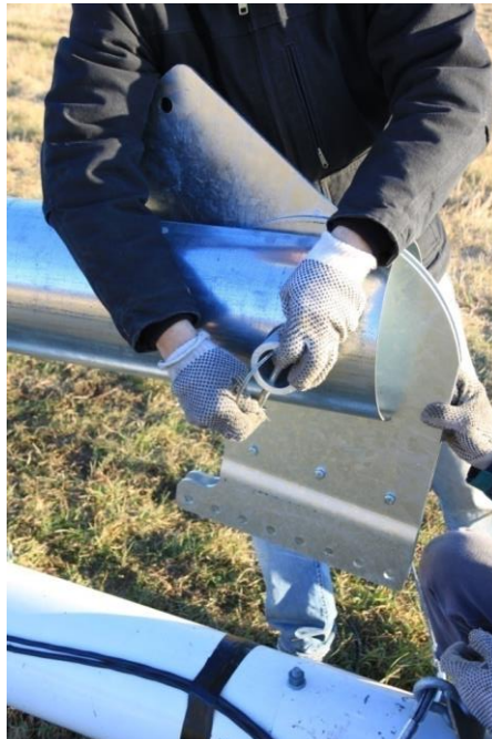
Picture 3-56: Secure ginpole rocker plate pivot pipe
