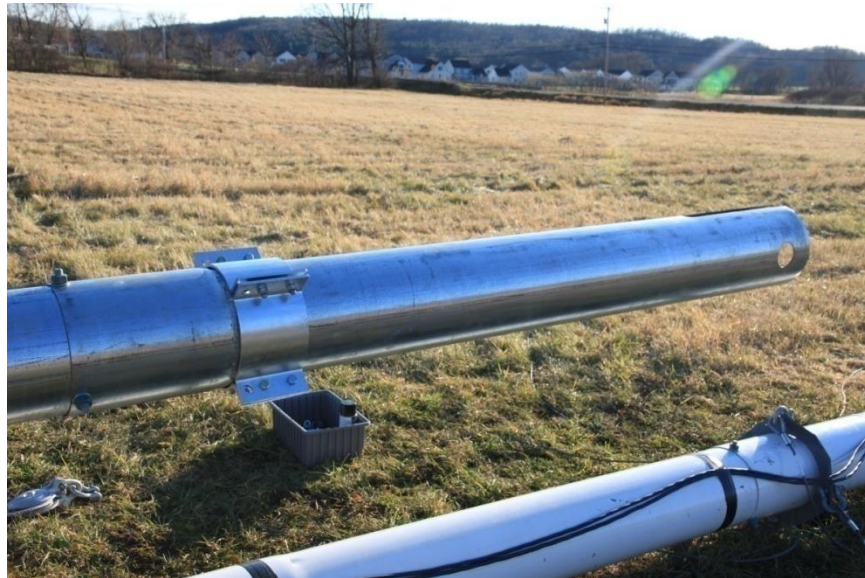
Picture 3-42: Ginpole jumper strut end-flange
