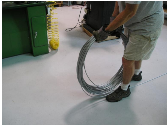
Picture 3-31: Unroll guy wires CORRECT
