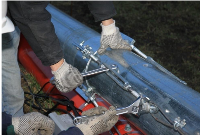
Picture 3-80: Tightening turnbuckles
