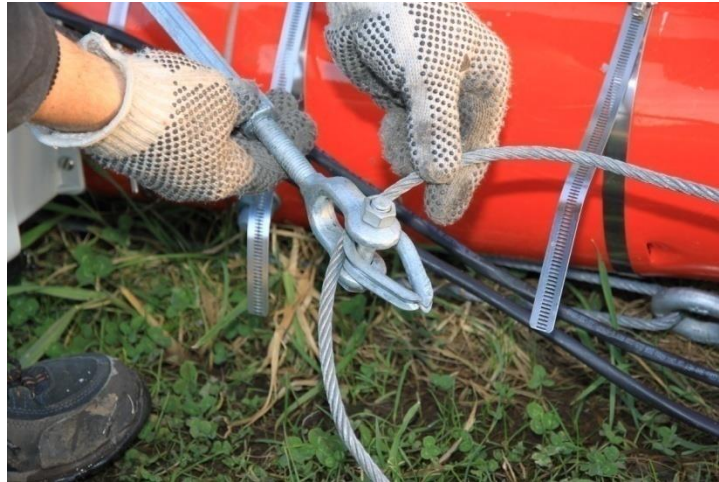
Picture 3-53: Attach jumper strut cable to turnbuckle
