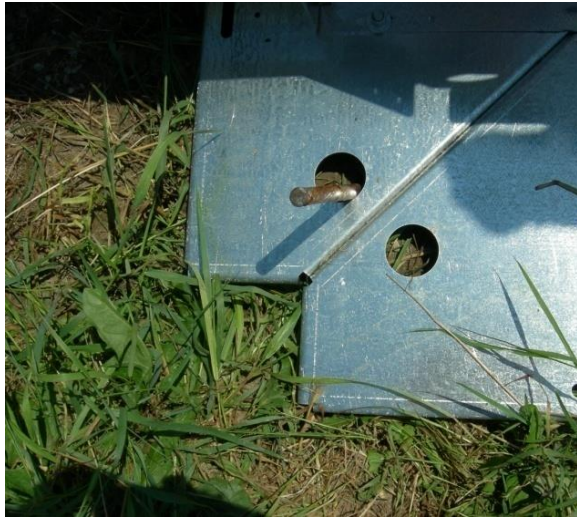
Picture 3-12: Ground Rod Placement
