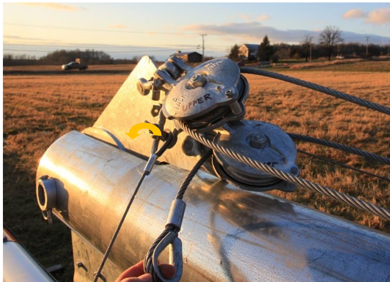
Picture 3-76: Reeving through pulley #4
