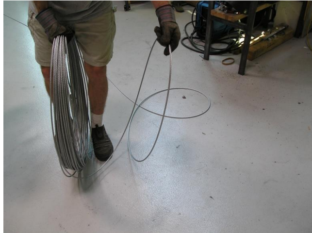
Picture 3-32: Unroll guy wires Incorrect!
