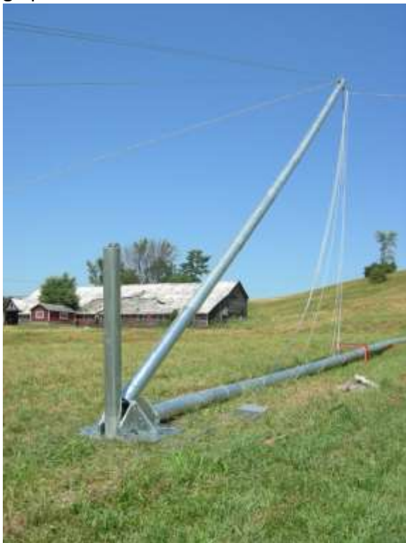
Picture 4-1: Ginpole tilt-up, Helper ginpole attached
