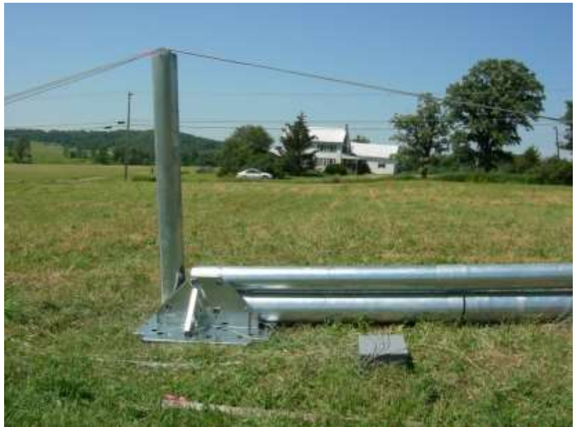
Picture 3-40: Winch cable over helper ginpole
