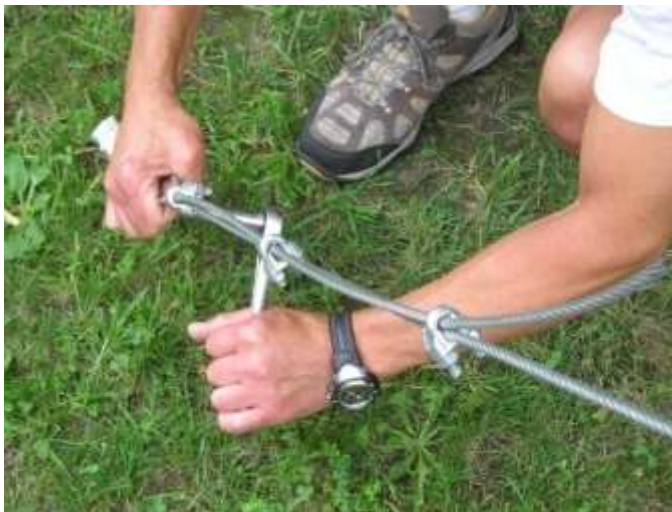
Picture 4-8: Loosen bottom 2 clips
