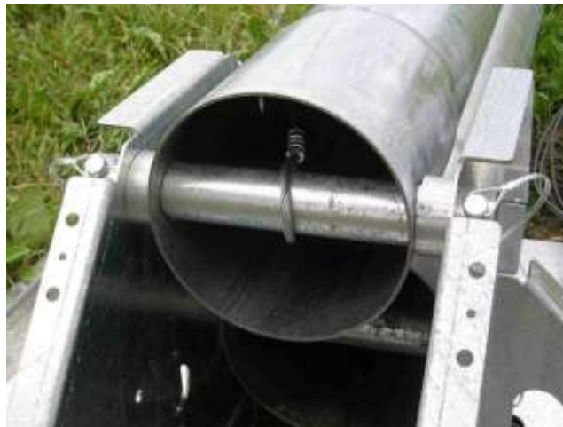
Picture 3-24: Attach ginpole base tube and safety cable
