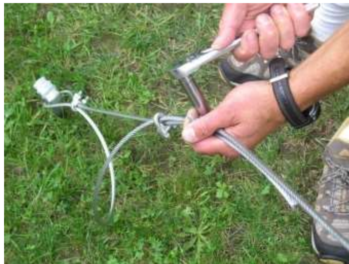
Picture 4-5: Re-tighten top clips before loosening bottom
