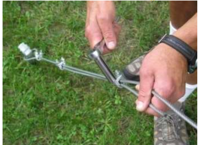
Picture 4-11: pull tail to remove loop, Re-tighten top clips
