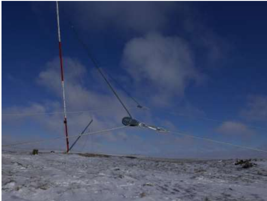
Picture R-4: Leader cables attached to back guywires using pulleys
