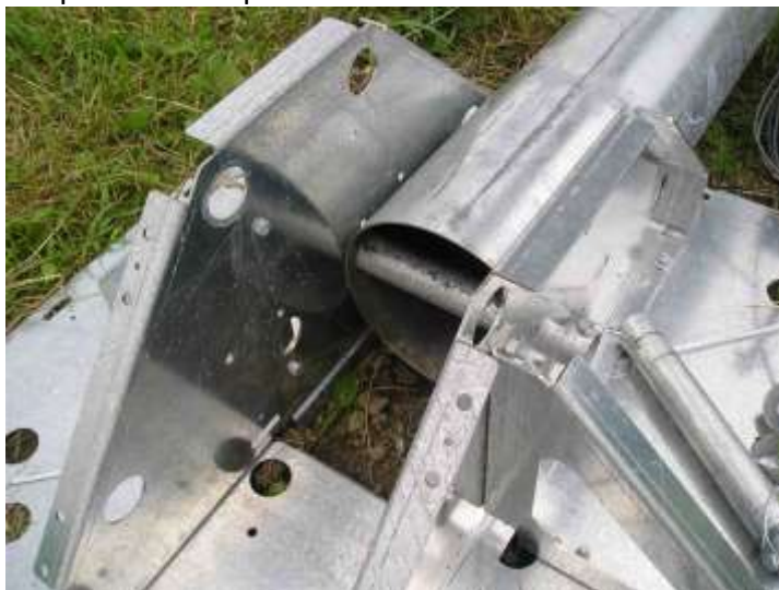
Picture 3-12: Baseplate assembly
