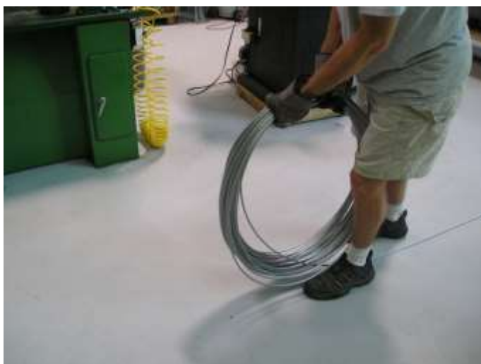
Picture 3-18: Roll out guy wire-Correct
