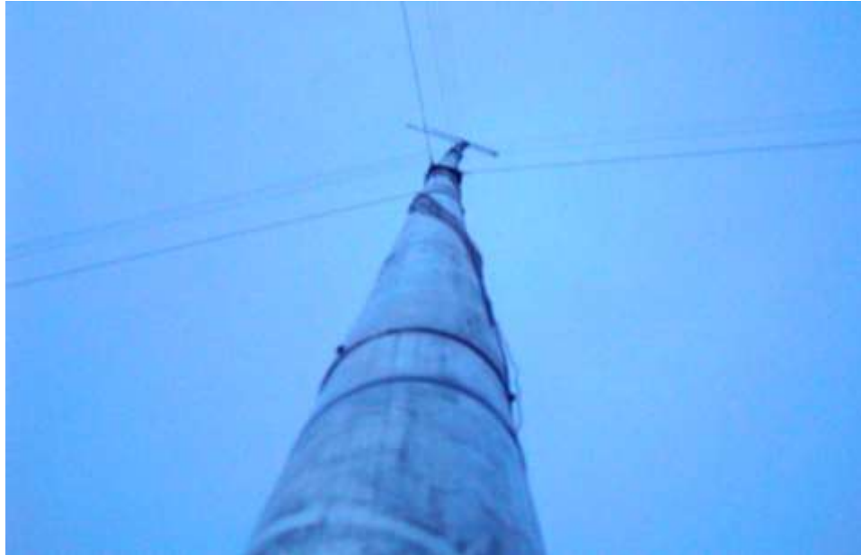
Picture 4-18: Plumb & Straighten
