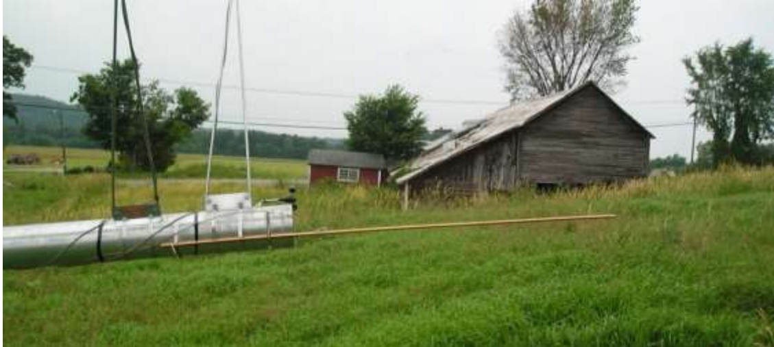
Picture 3-14: Lightning rod attachment
