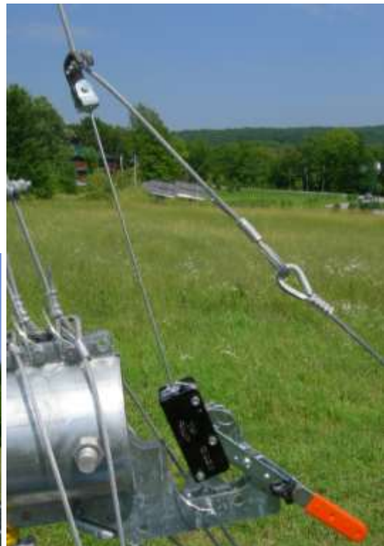
Picture 4-17: Remove hoist claw
