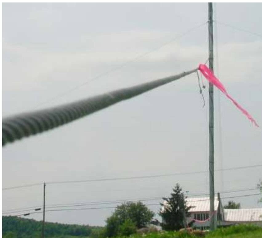
Picture 4-19: Level 1 Guy, Sag = 1.2 Tube (Acceptable)
