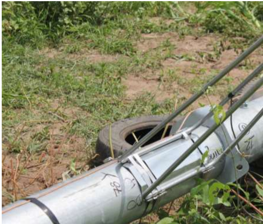
Picture 3-16: Hose clamp booms to tower
