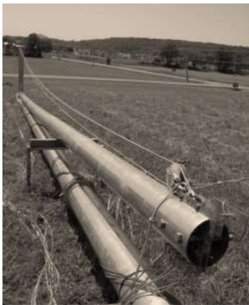
Picture 3-39: Winch cable wound on pulleys
