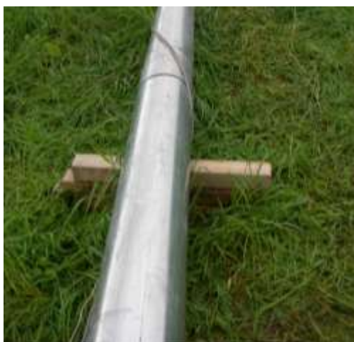
Picture 3-13: tower assembly support
