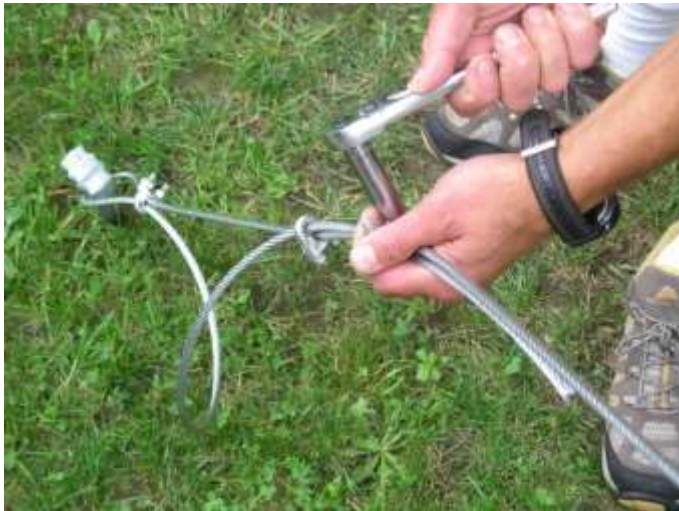
Picture 4-10: Loosen top clip
