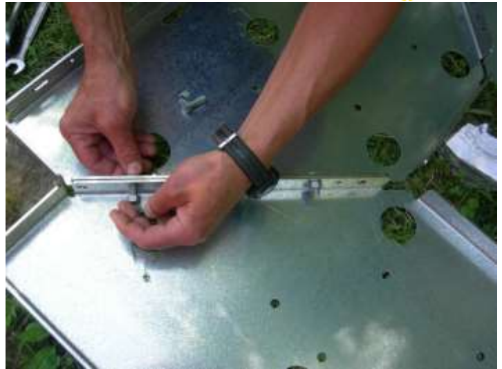
Picture 3-2: Baseplate assembly
