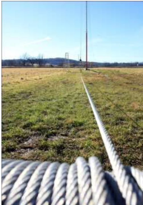
Picture S-5: Correct winch cable fleet angle
