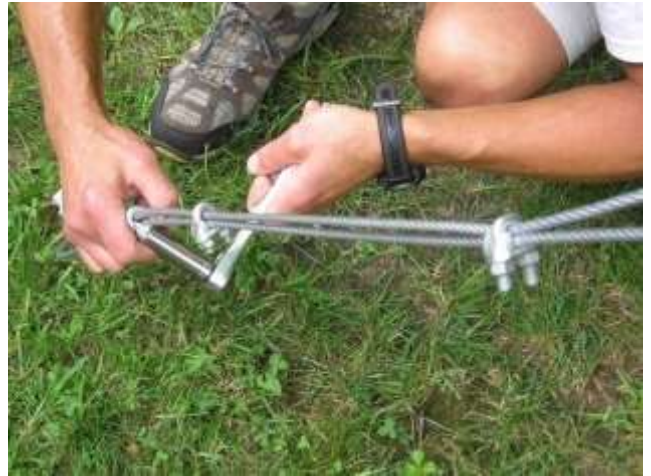
Picture 4-7: Re-tighten bottom slip when slack is gone
