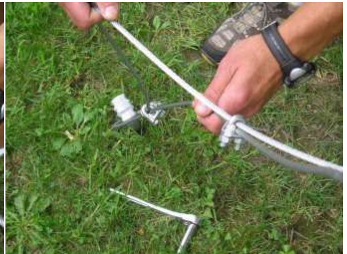
Picture 4-4: pull slack into line (make a loop)
