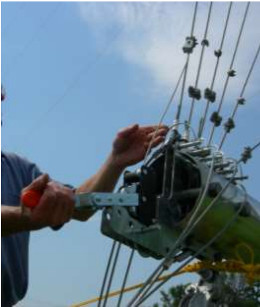
Picture 4-14 & Picture 4-15: use hoist to loosen lifter to remove from ginpole
