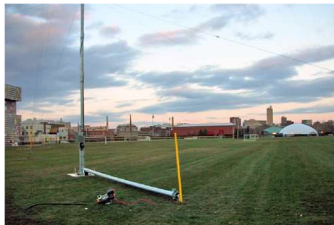
Picture 4-20: Guy Guard on winch anchor
