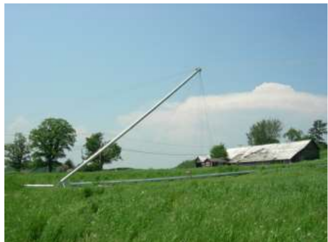
Picture 4-2: Ginpole high enough to remove helper ginpole
